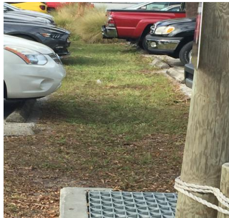
Figure 2.2 Grass parking swale demonstrating the LID construction configuration to filter parking lot stormwater (picture used with permission from Rushton & Hastings, 2001)
